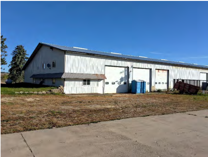
View of the barn proposed for renovation.
